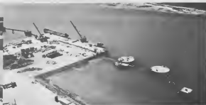
Pier nearly completed in January 1970, built by Netherlands Harbour Works Company.
